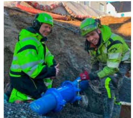
*"The Supa One™ coupling is very easy to install. Tightening with a standard power tool and torque wrench to 150 Nm works very well."* - Kaare Mortensen A/S, Norwegian construction company.
